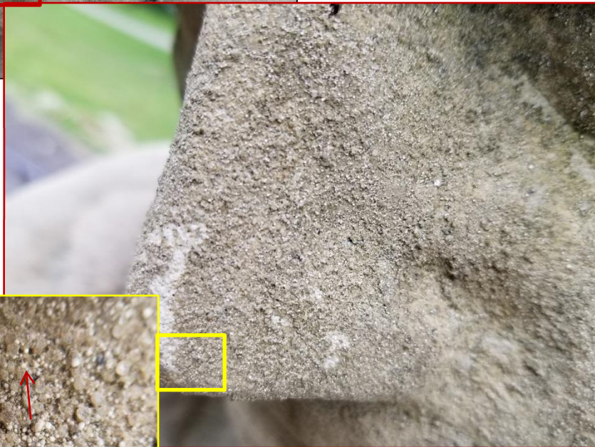
Photo 17, right: Detail of Photo 16.
